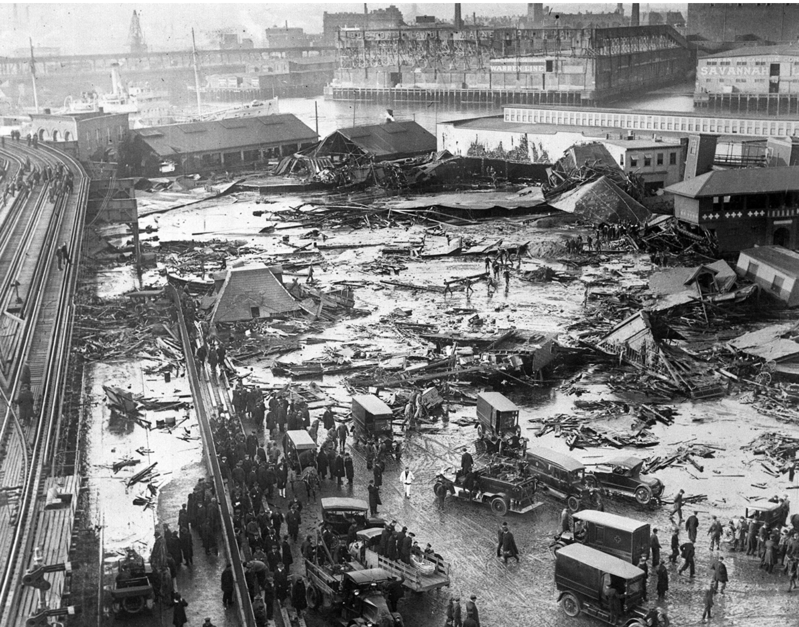
The sticky tidal wave swept away buildings, people, horses, damaged the elevated railway (at left) and demolished the North End market (above) before oozing into the inner harbour. Photo: Boston Library
